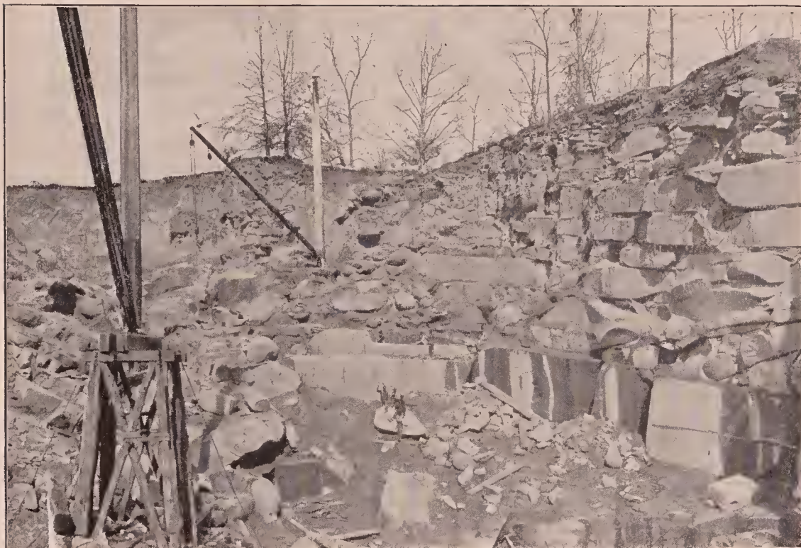
FIG. 1.—GRANITE QUARRY NEAR WOODSTOCK, BALTIMORE COUNTY.
